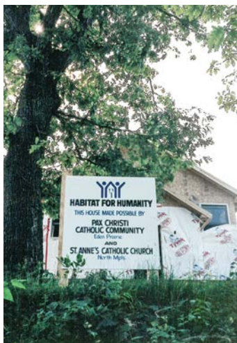
Pax Christi's ten year anniversary Habitat for Humanity project.
